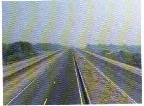
Janjira Approach Road Tree plantation at Approach Road
