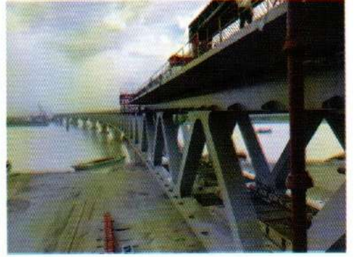
Road slab Erection
