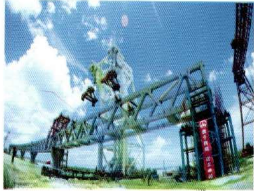
Span erection
