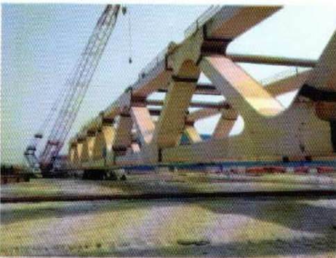
Truss Assembling
